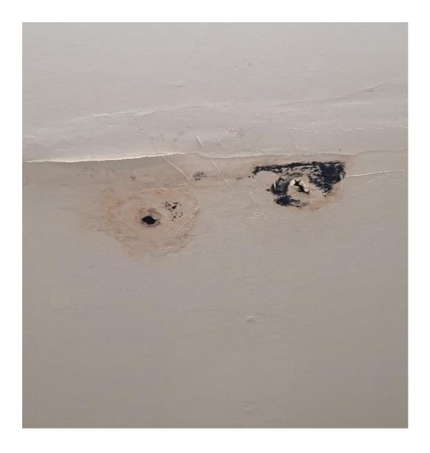
Bathroom Ceiling leaking with mold
