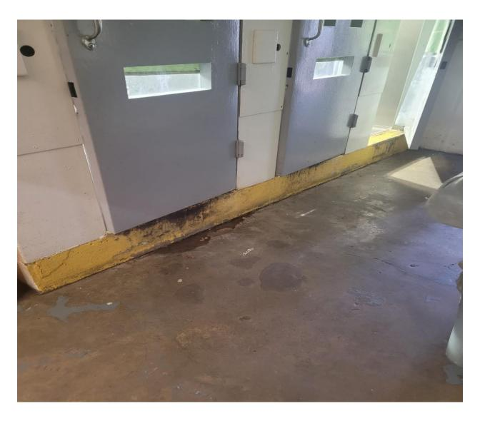
Water leaking from underneath the wall
