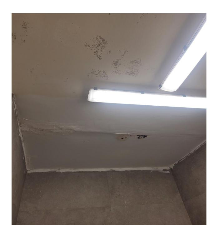
Bathroom ceiling leaking water
