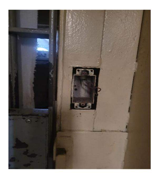
Exposed electrical wires from light fixture
