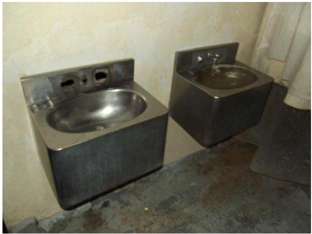
Unit 29F, B-Zone 1<sup>st</sup> Lavatory sink is missing knobs and 2<sup>nd</sup> sink is stopped up
