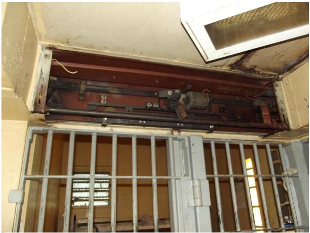
Unit 29G, B-Zone Panel cover is missing above the cell doors
