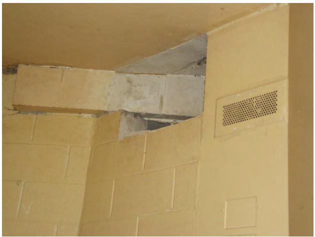
Unit 29G, B-Zone Concrete blocks are missing from the top wall
