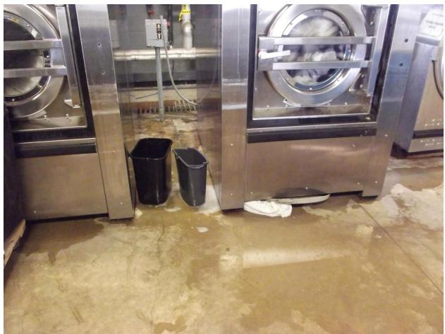
Unit 32 (Laundry) 2<sup>nd</sup> machine leaks water from underneath
