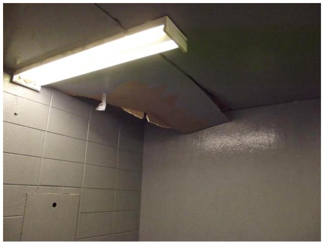
GYM bathroom ceiling is falling down
