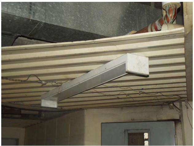
Unit 29B Ceiling has exposed wires and light is out
