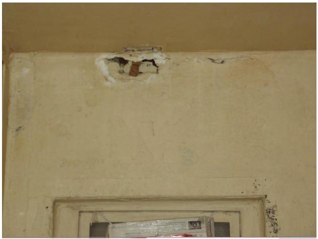
Unit 29G, B-Zone Cell #71 ceiling has a hole and leaks water
