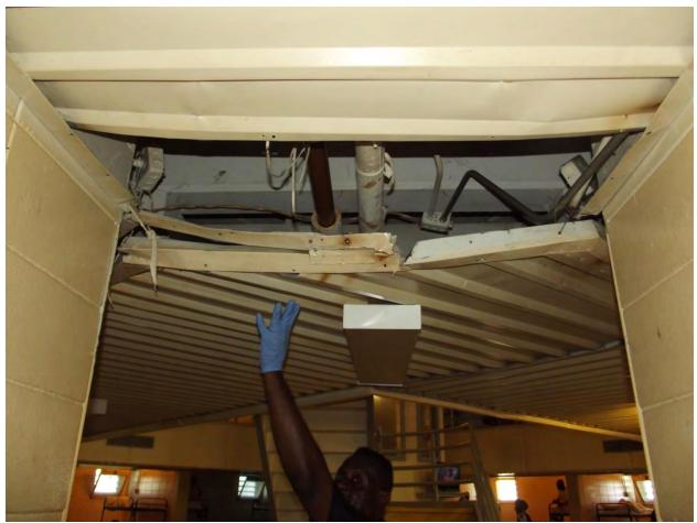
Unit 29E, A-Zone Ceiling Frame is Broken
