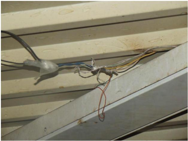
Unit 29B ceiling has exposed wires
