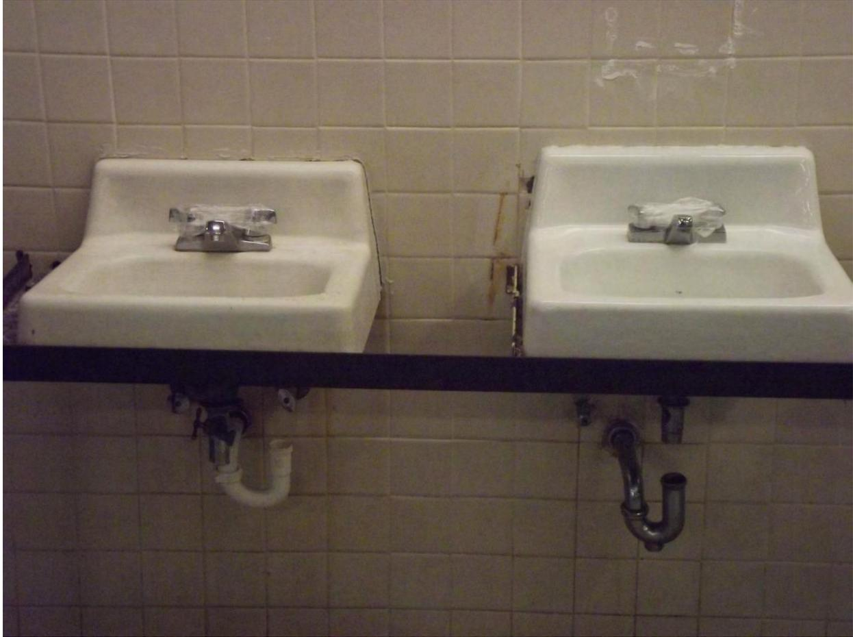
**Unit 30B Zone A – 2<sup>nd</sup> and 3<sup>rd</sup> lavatory sinks are missing pipes**
