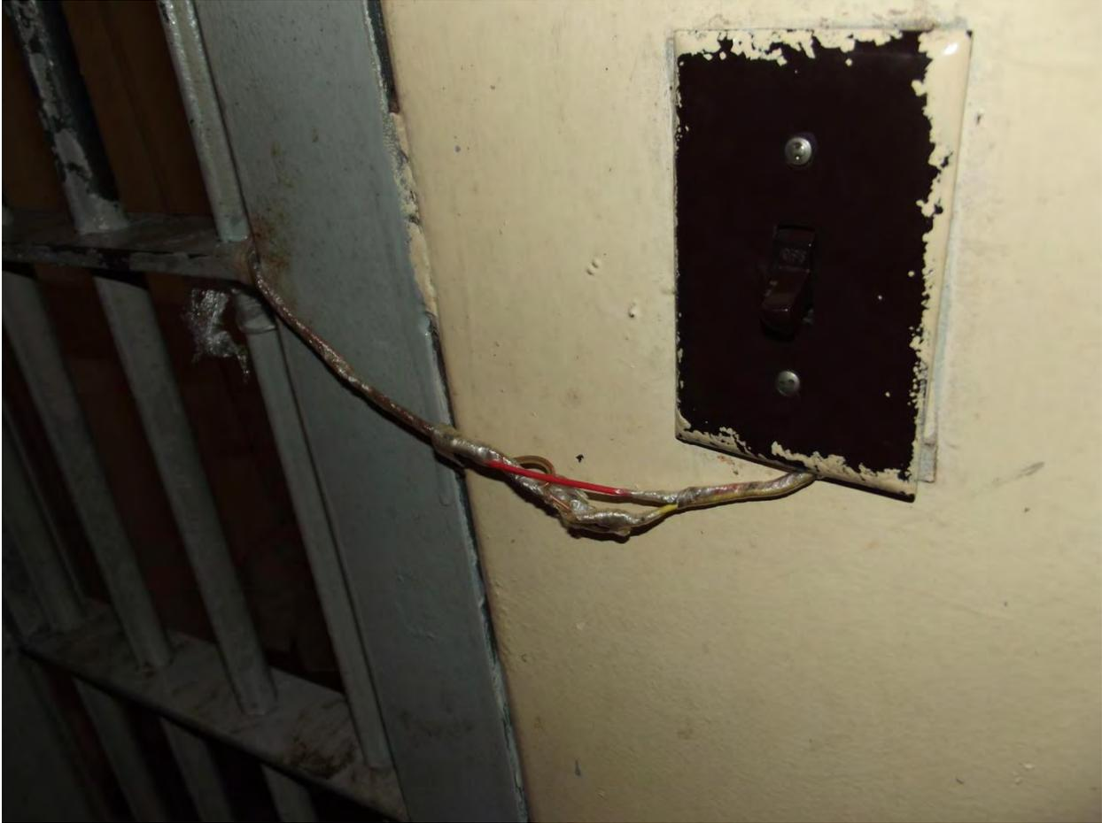
**Unit 29H, B-Zone cell has exposed wires running from switch box**
