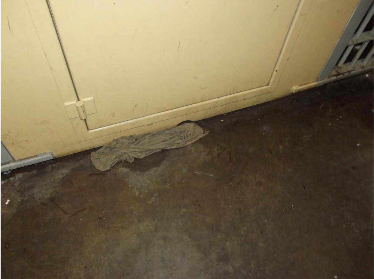
**Unit 29G, B-Zone Cell #14 – water leaks from the cell into the Corridor**
