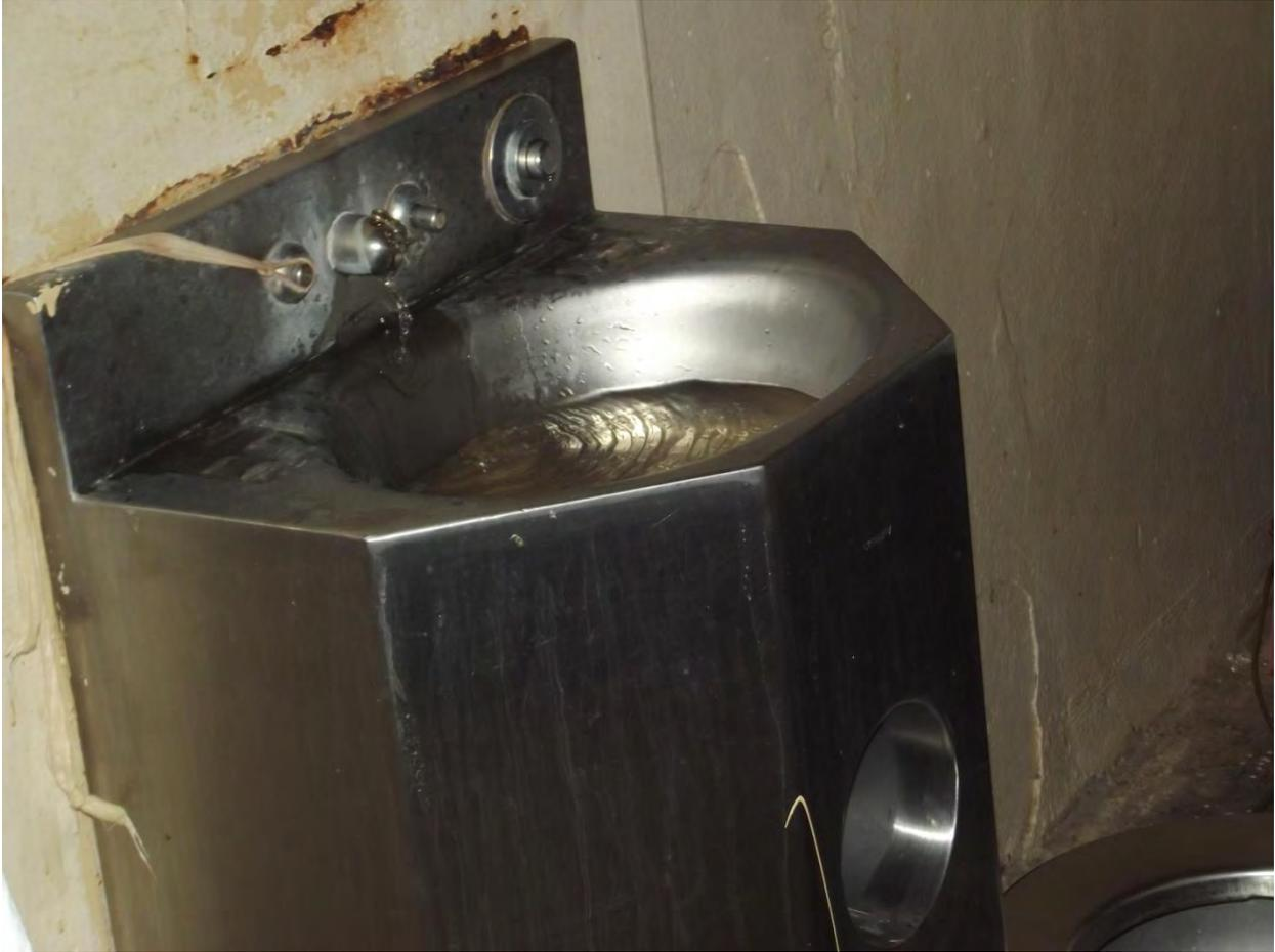
**Unit 29G, B-Zone Cell #34 lavatory sink is stopped up and water runs continuously**
